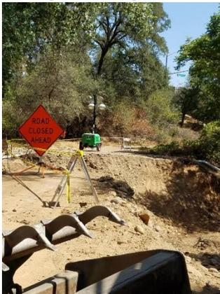
**Hinkle Creek Culvert** - Contractors are in the process of repairing a culvert that washed out from storm water three years ago in the Negro Bar Unit of the State Park. The culvert allowed the creek to flow under a road, which later served as a paved multi-use trail. Creek water is being diverted during construction.
